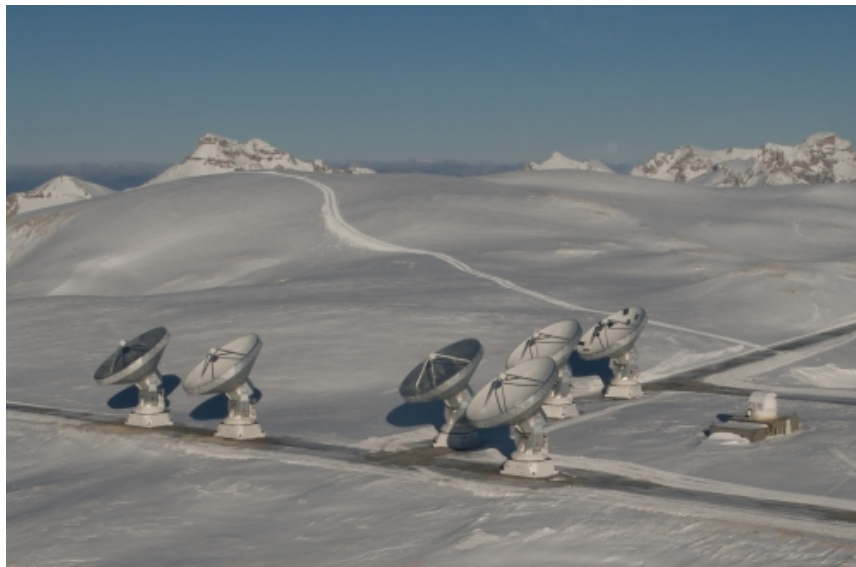
Figure 1.4: The NOEMA interferometer in compact configuration, before the upgrade which will increase the number of antennas from 6 to 12. Image adopted from IRAM website.
